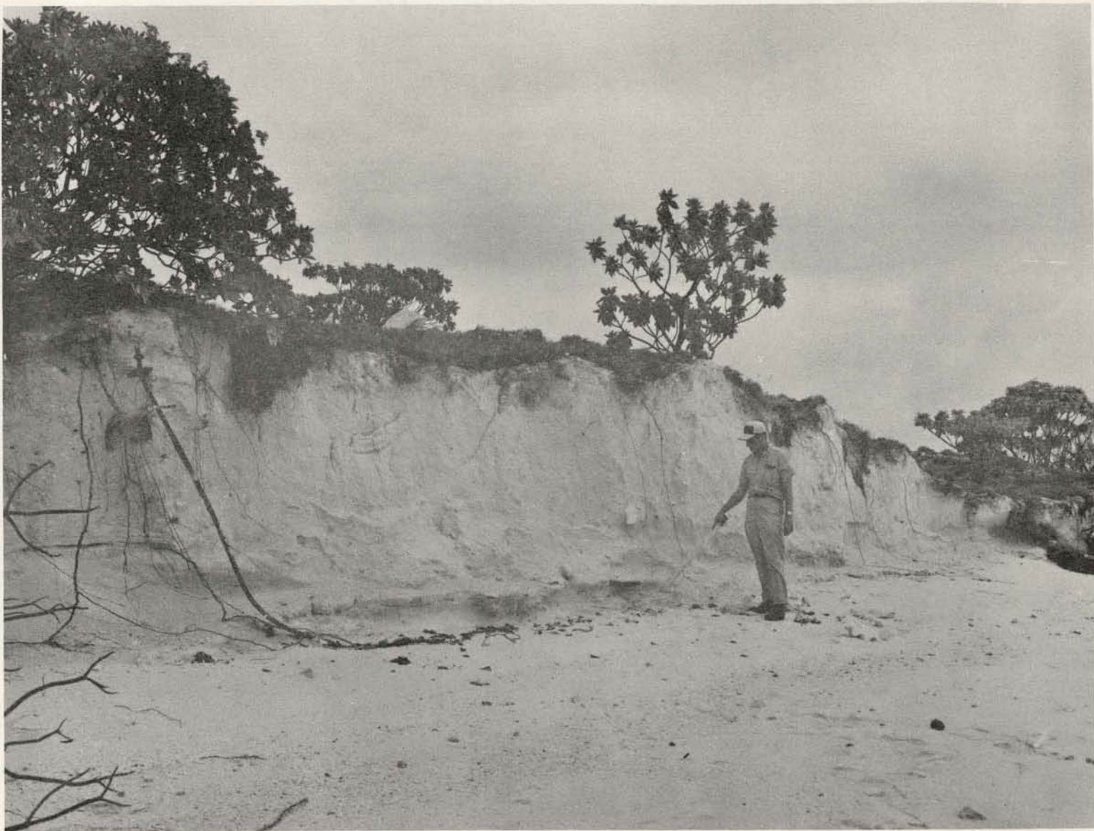
Fig. 46. 1964 photograph showing shore erosion at north end of Irene island. Note wave undercutting taking place.
